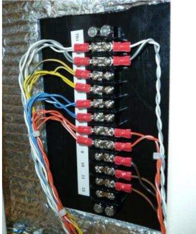
TB1, 12 Position, Dual Row, #6 Screw Terminals Signal Wire Interface and Take-Off
