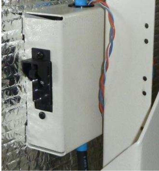
Battery Breaker 60 Amp with Finger Guard
