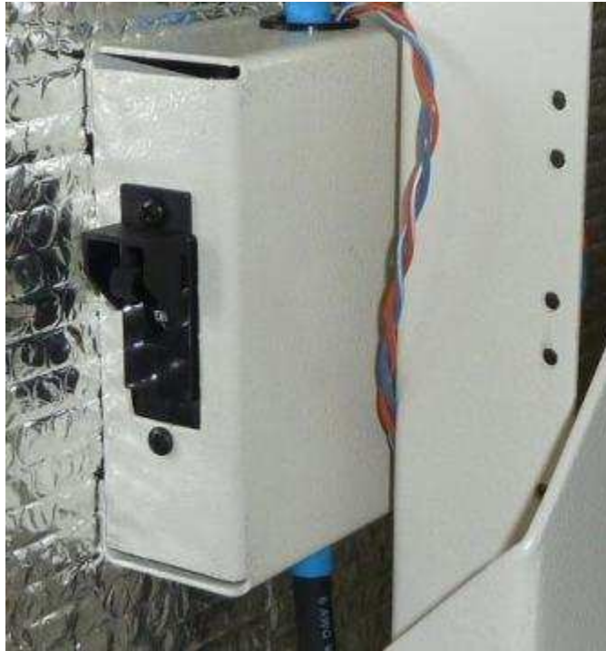
Battery Breaker 60 Amp with Finger Guard
